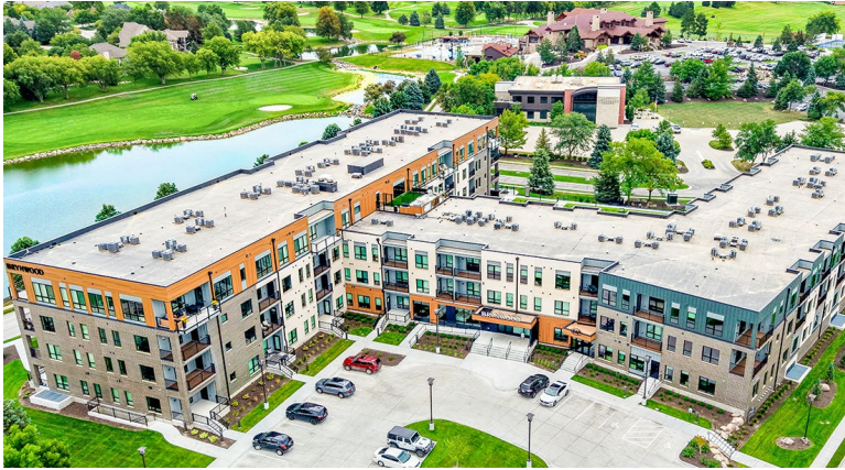
Brester Construction Brynwood at Wilderness Ridge
