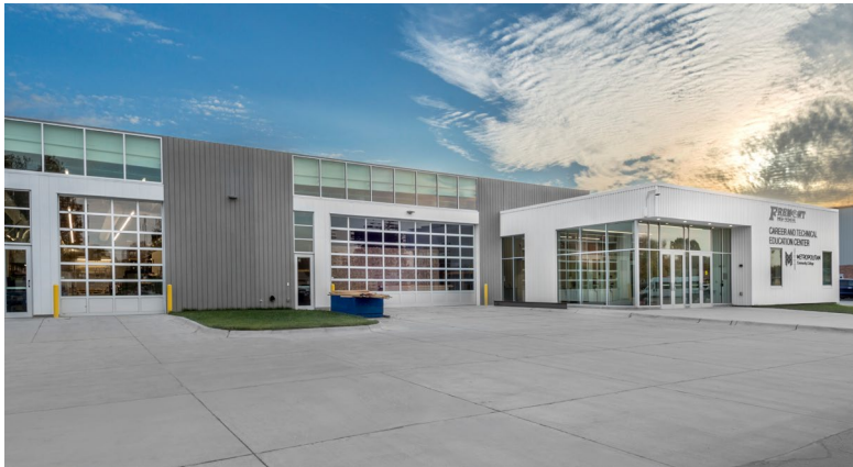
Hausmann Construction Fremont Public Schools, Fremont High School
