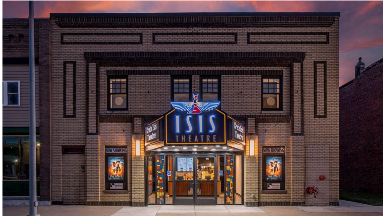
Kingery Construction Co. Isis Theatre
