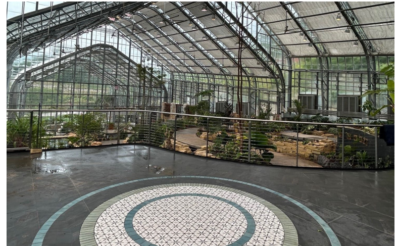
Kiewit Building Group Inc. Lauritzen Gardens Conservatory Renovation
