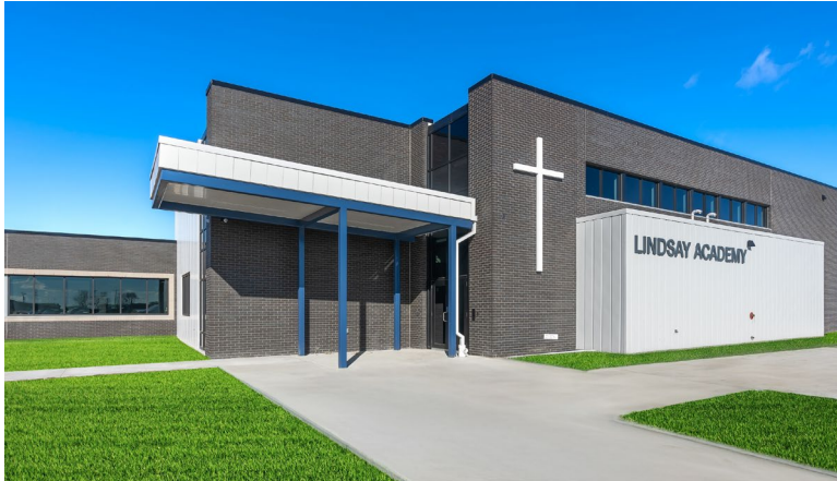
Sampson Construction Co., Inc. Lindsay Academy High School
