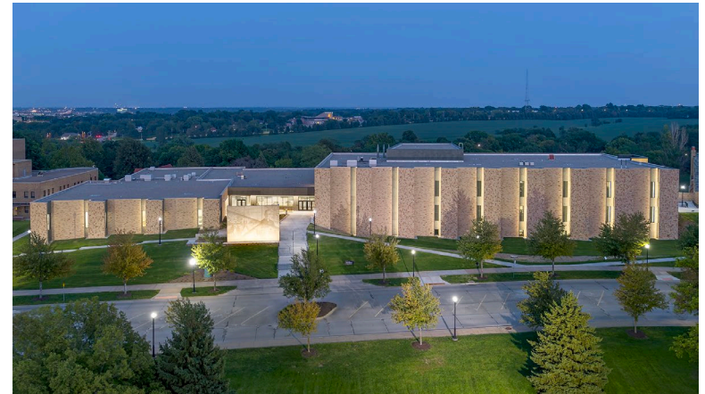
MCL Construction Boys Town Education Center
